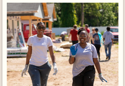
Sea Island volunteers helping at the Habitat for Humanity build site.
